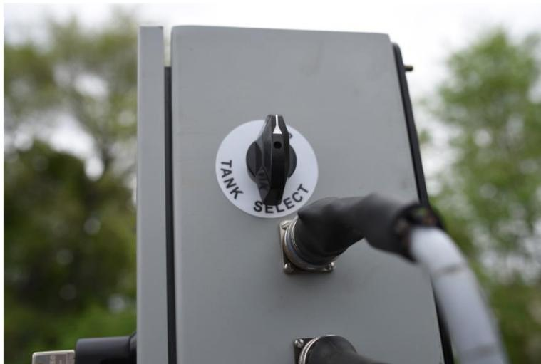
**Figure 28:** Tank select switch
