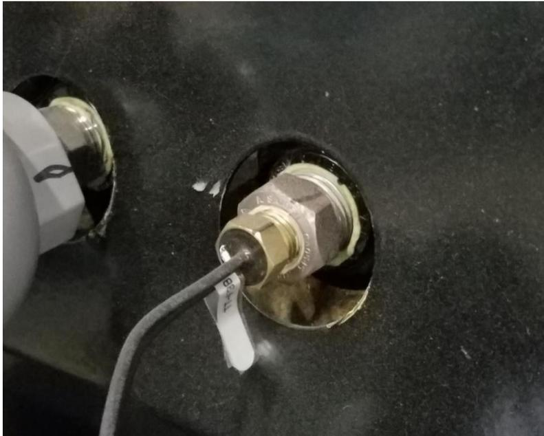
**Figure 24:** Emulsion tank over-temperature switch.
